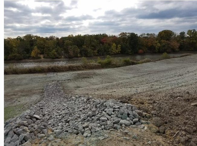
View: Phase III Rip Rap Channel
