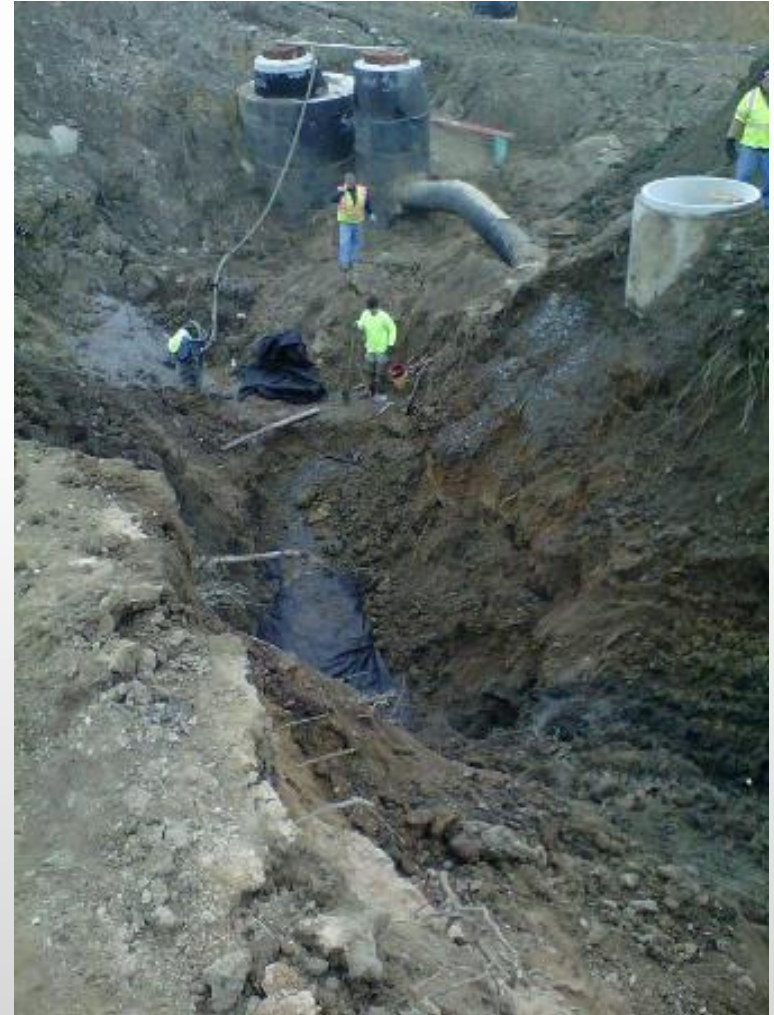
View: Underdrain for Cutoff Wall
