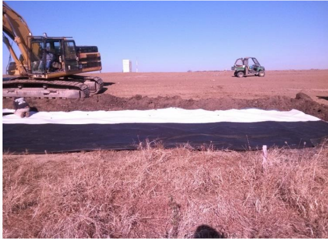
View: Phase I Lined Swales
