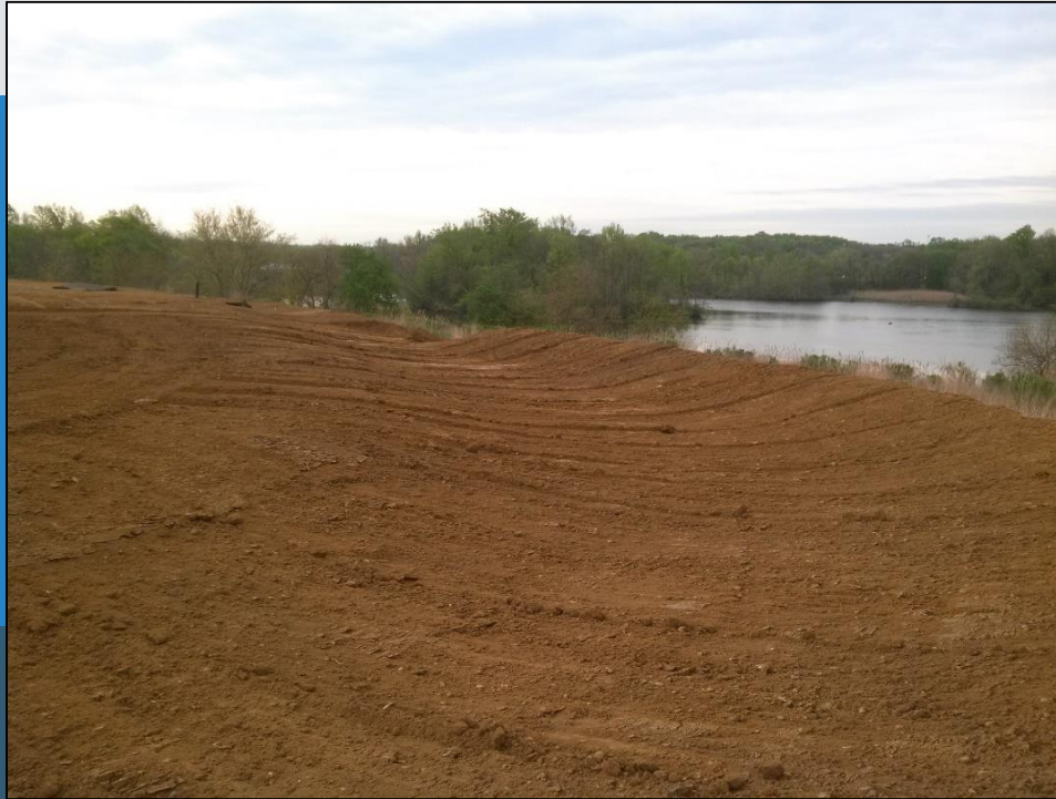
View: Phase I Berms, Lined Swales prior to seeding
