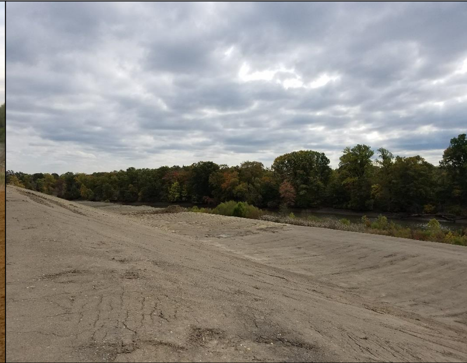
View: Phase III Berm and swale system prior to seeding
