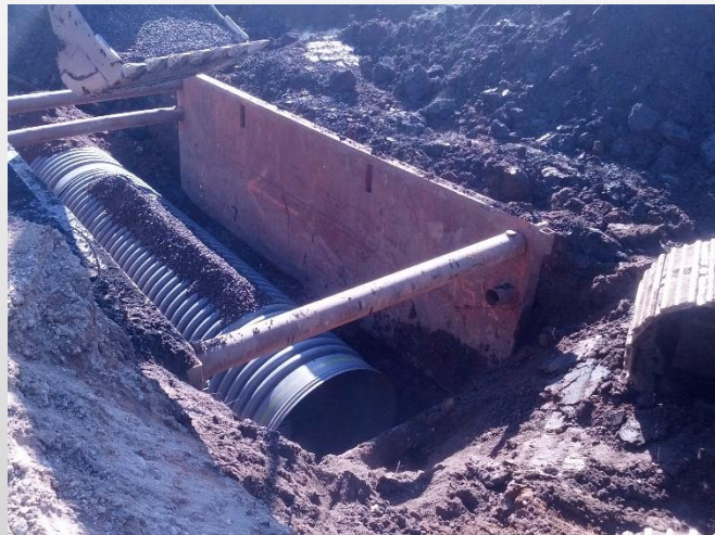
View: Upgradient Stormwater Pipe
